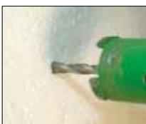
1. Drill a hole in the insulation.
