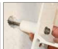
5. For push-through installation: Install the bracket with RECA Dimos.
