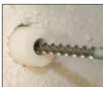
2. Drill a hole in the substrate (use RECA Dimos as a centering aid if necessary).
